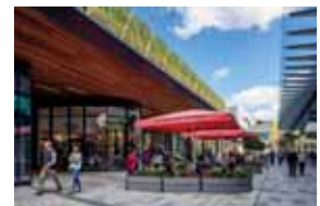
Commercial development including food, drink, retail, entertainment with 3 floors of use above (eg. cinema, apartments, offices)
